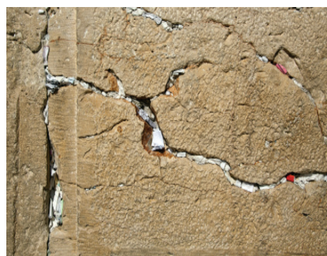
Notes in the cracks of the Temple wall
